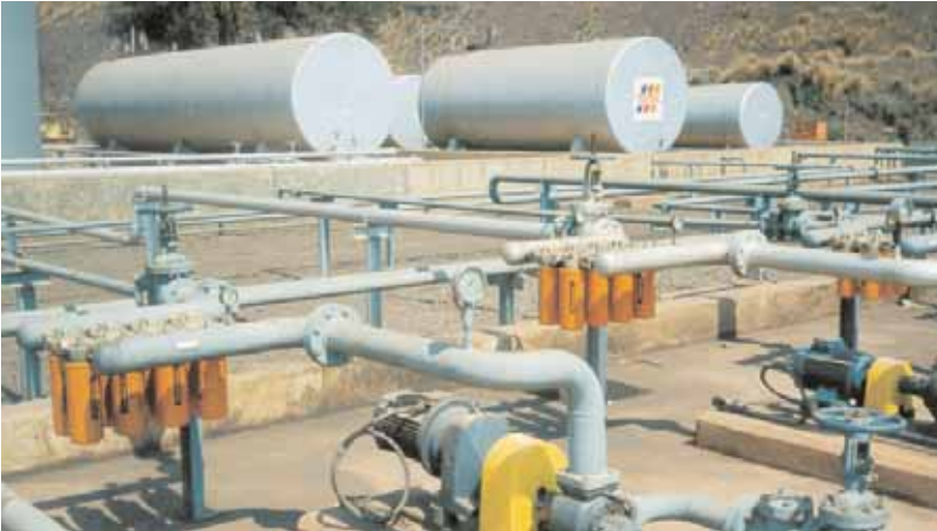
Donaldson Duramax units at this South Africa ore mine filter bulk oil as it runs from storage tanks to delivery trucks for transport to the customer. This parallel filter configuration provides for high flow rates.
